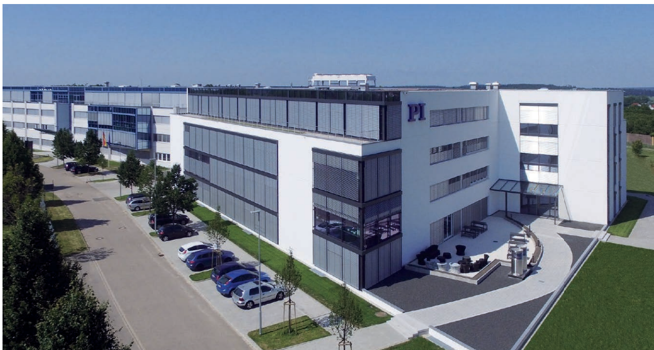
The PI headquarters in Karlsruhe, Germany, manifests the continuous growth. In front, the 2017 Technology Center
