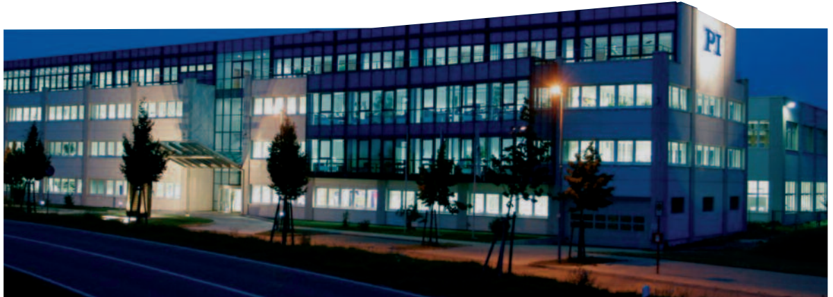
PI headquarters in Karlsruhe
